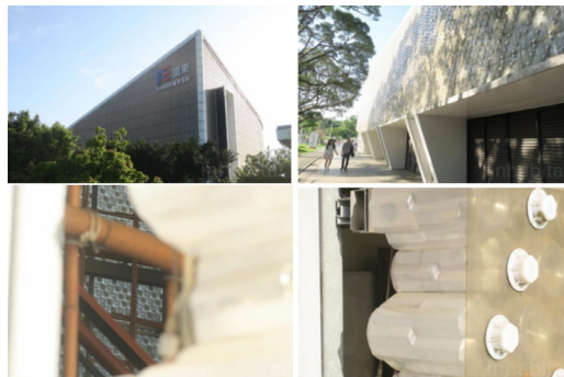
Gambar 14. Tampak bangunan dan struktur dinding botol plastik daur ulang (Sumber: https://inhabitat.com/amazing-plastic-bottle-architecture-withstands-earthquakes-in-taipei/ )
