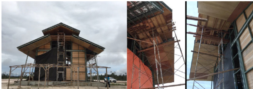
Figure 5 Construction process of Oikumene Church, Sajau Project.
