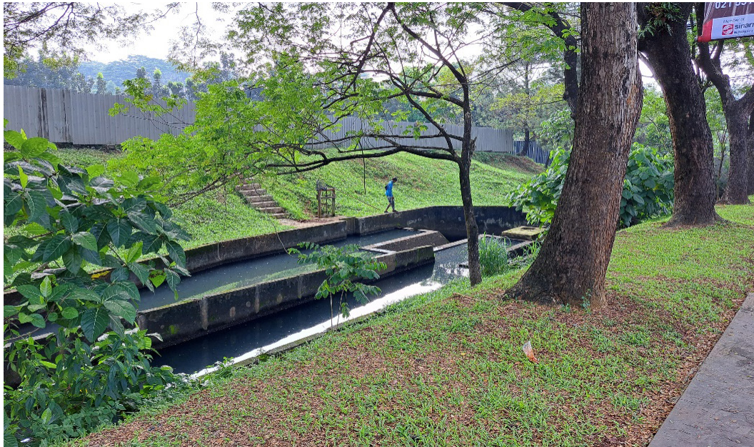
Image 3 Waste Water Drainage. (Source: Researcher, 2024)
