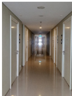
Image 12 The existing condition of BB Apartment Corridor (Source: Author's Documentation)
