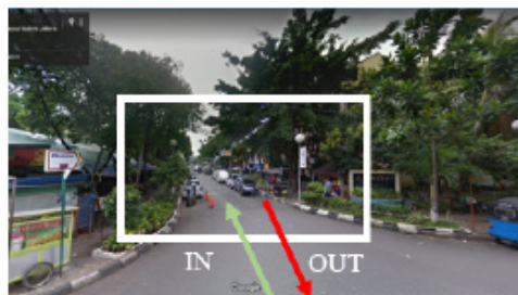
Image 3 The Main Gate of the Rusun Apron Kemayoran. The condition of the main gate of the Apron Flat since it was built until before the parking gate was built, only uses a portal and can be accessed by anyone. (Source: Google Streetview 2019)
