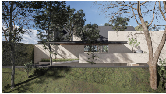
Image 5. Facade, GGT House Source: Document of SS (2021)
