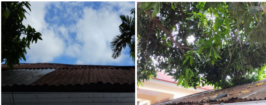
Figure 2. The condition of the roof prior to cleaning
